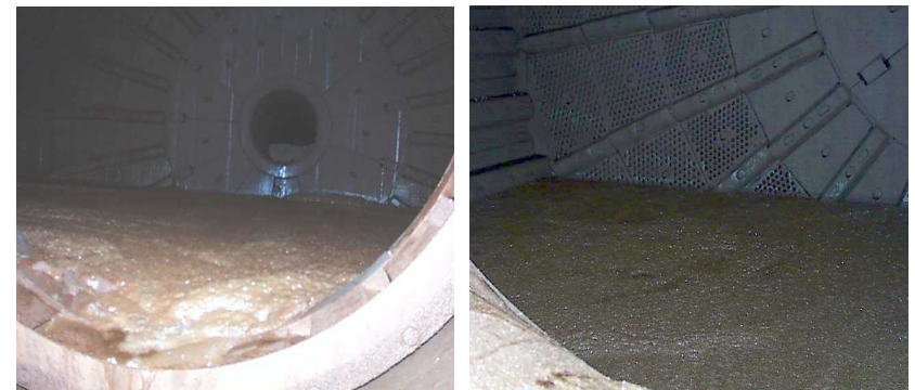
Figure 7: Crash Stop Charge Pre (left) and Post (right) Installation at 390tph
