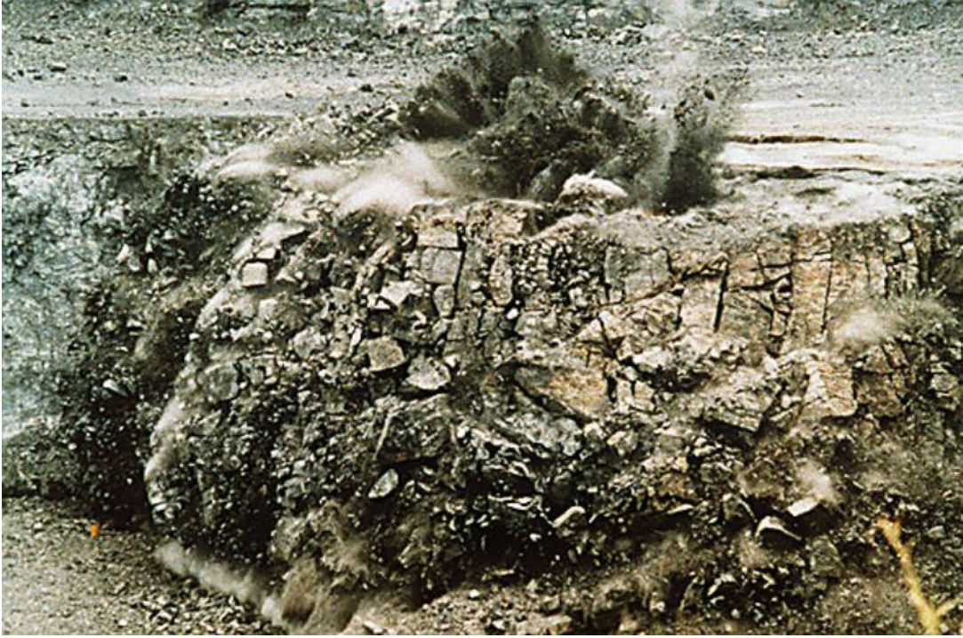
Figure 8 – Picture of Free Face During Blasting
