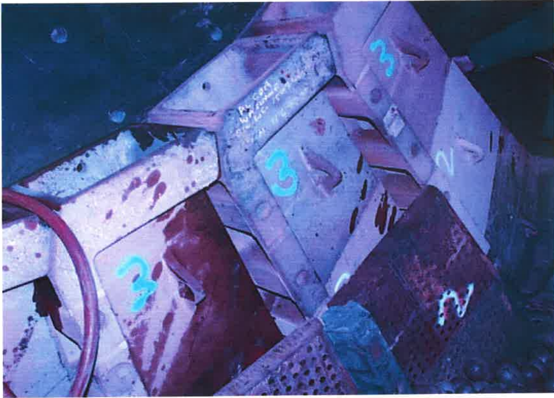
Figure 12 – Twin Chamber Pulp Lifter Installation
